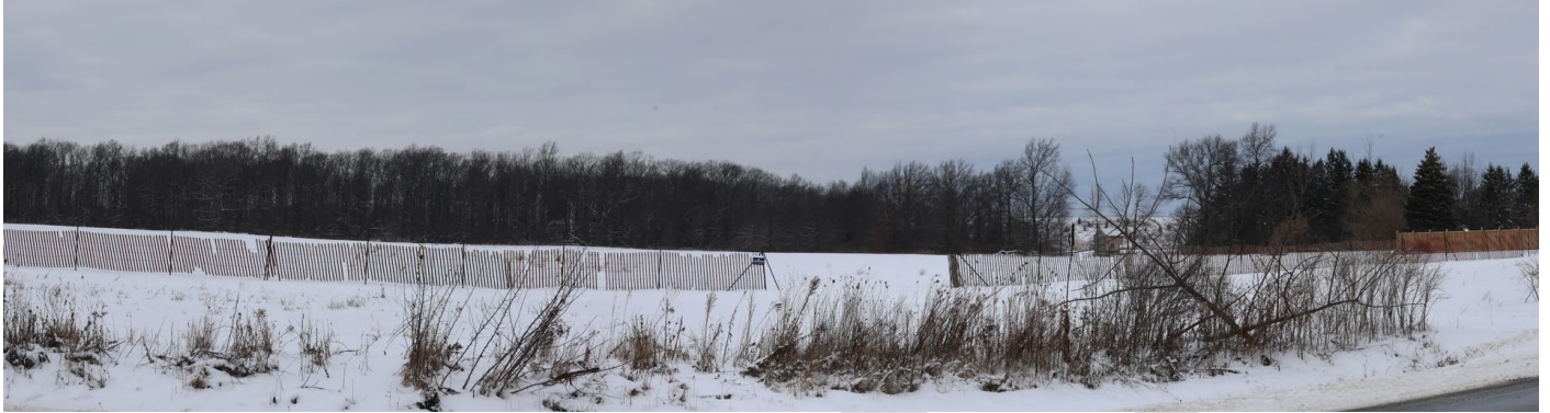
Photo 16 Photo Location 27 – Existing Condition
