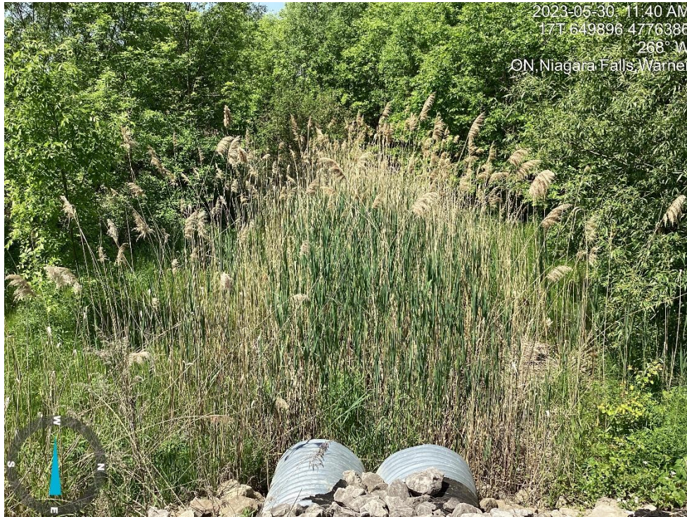
Photo 27 May 30, 2023. Reach 2. View of road crossing facing west.
