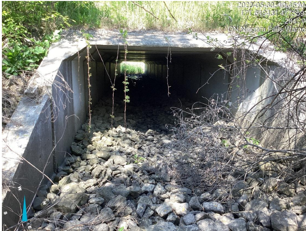
Photo 23 May 30, 2023. Reach 1. View of culvert under Beechwood Road. Photo facing west.
