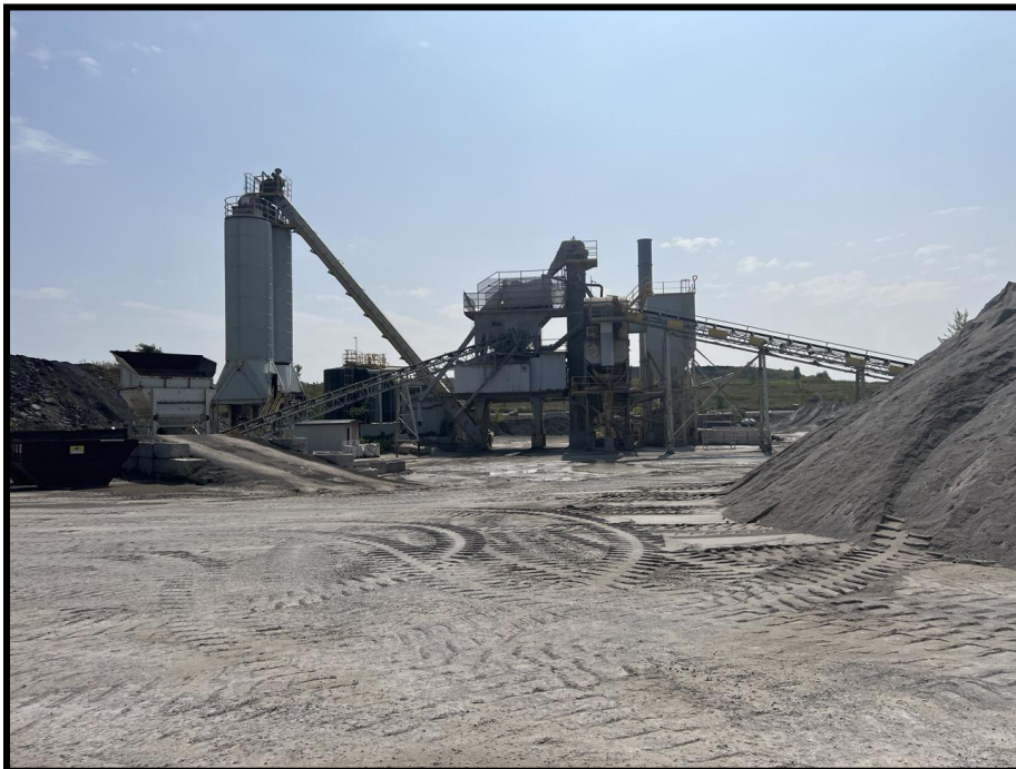
Image 4: Disturbed Lands (September 5, 2025; Facing East)
