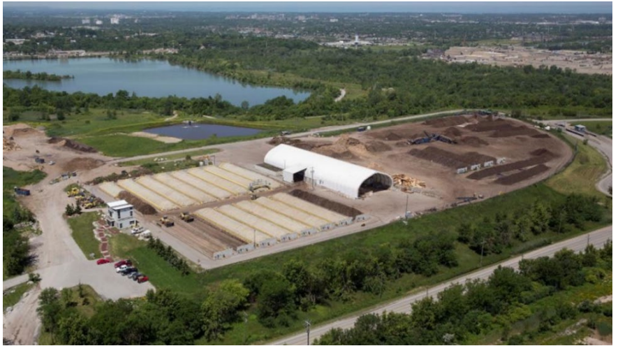
Figure 2.2 Walker's Niagara Composting Facility, Niagara, Ontario
