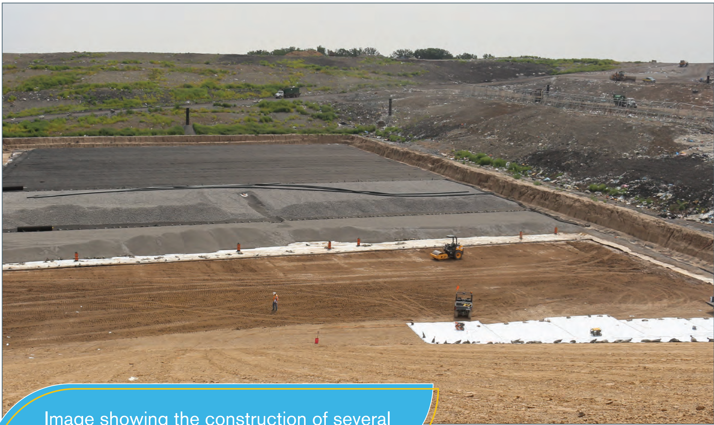
Image showing the construction of several layers of the engineered landfill liner
