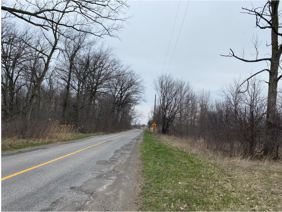
Photo 1 View of access road just west of BBS-23-07. Photo facing north and taken on April 11, 2023.
