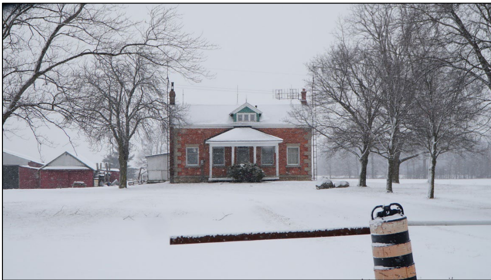
Photo of dwelling located at 8653 Thorold Stone Road (source: MHBC)
