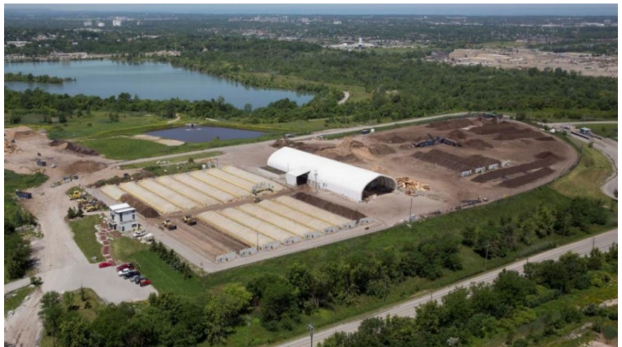
Figure 2.2 Walker's Niagara Composting Facility, Niagara, Ontario
