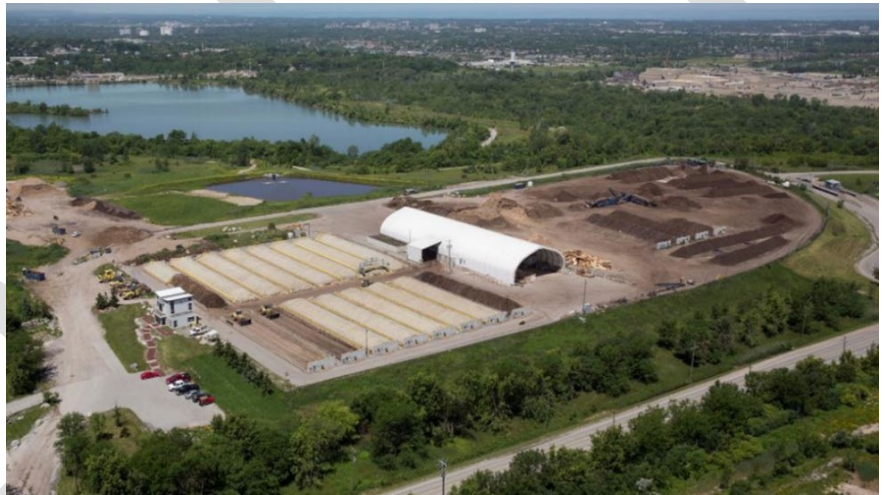
Figure 2.2 Walker's Niagara Composting Facility, Niagara, Ontario
